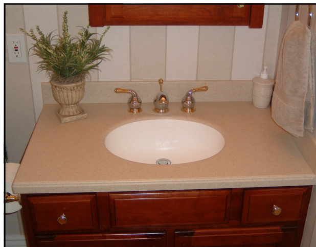
Acrylic Series Sink Installed in Solid Surface
